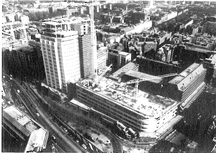
THE REDEVELOPMENT OF UNIVERSITY COLLEGE LONDON HOSPITAL
